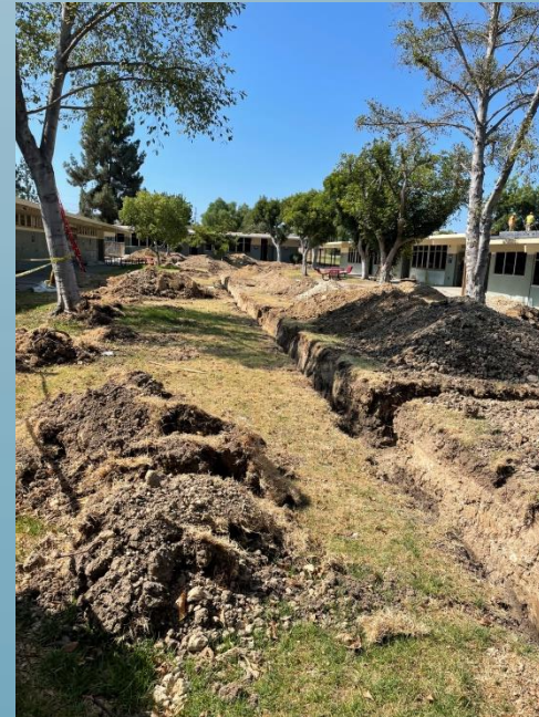
Storm Drain & Electrical
