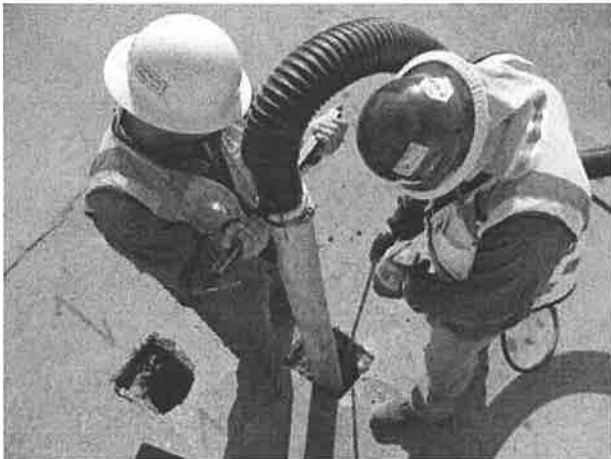
C Below technicians performing potholing
